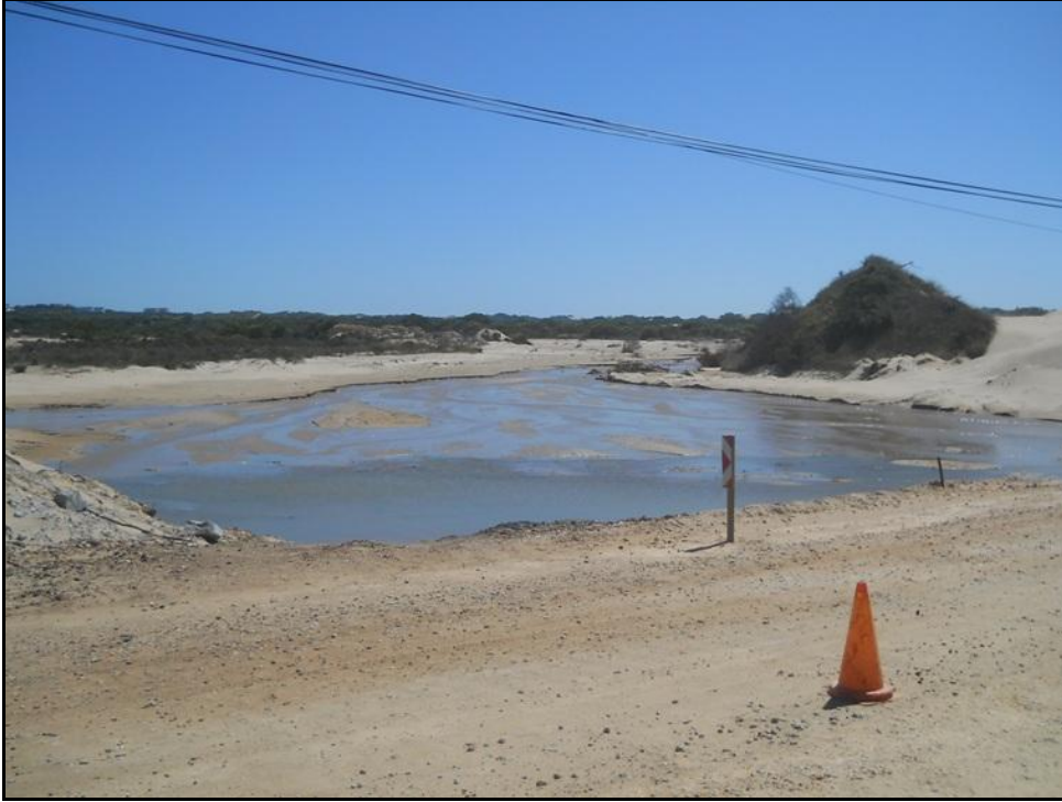
Figure 5: Upstream view of Sand River crossing.
