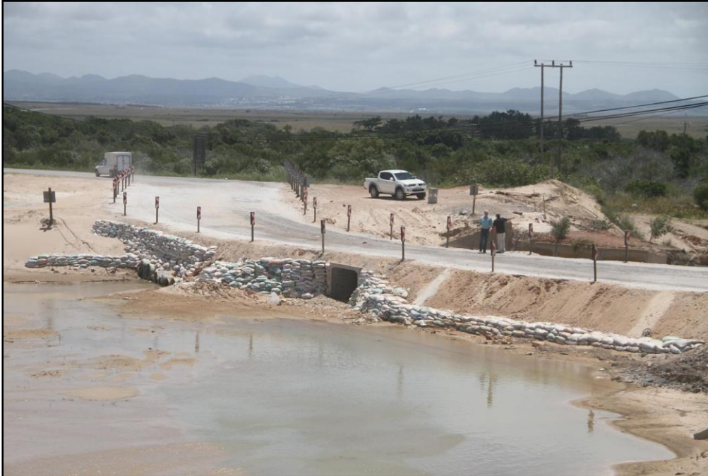
Figure 3: View of the current bypass and crossing over the Sand River.
