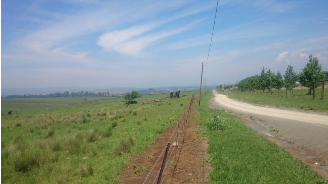
This photo shows the route of the sewer rising main along the existing road.
