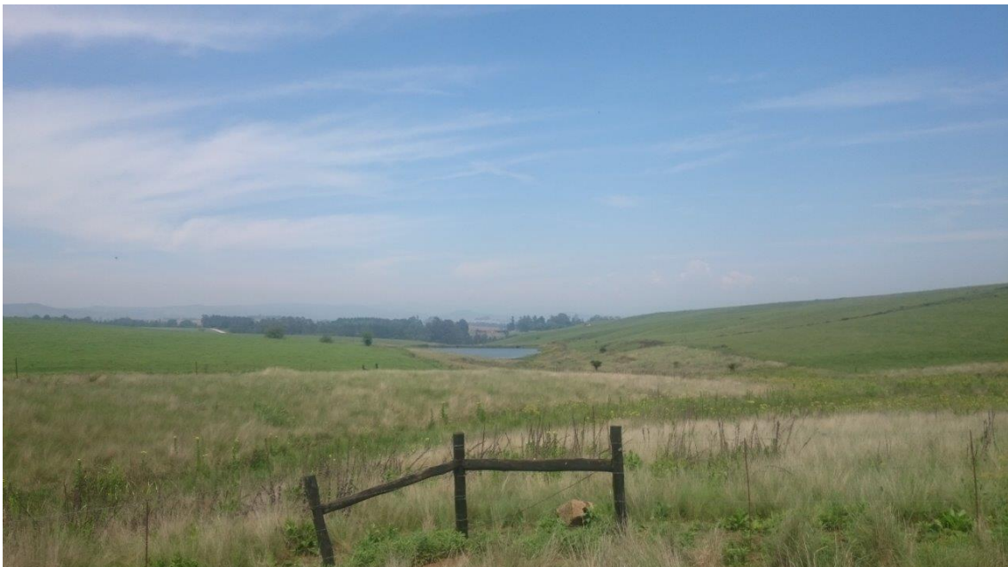
This photo shows the dam and wetland downstream of the land development area.
