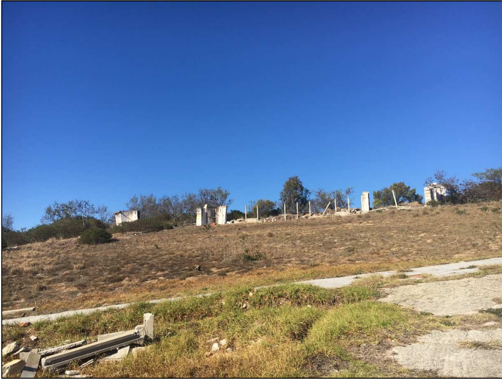
Photo 5: An example of the other structures on the site, previously associated with the stadium, which will be demolished as part of this project.
