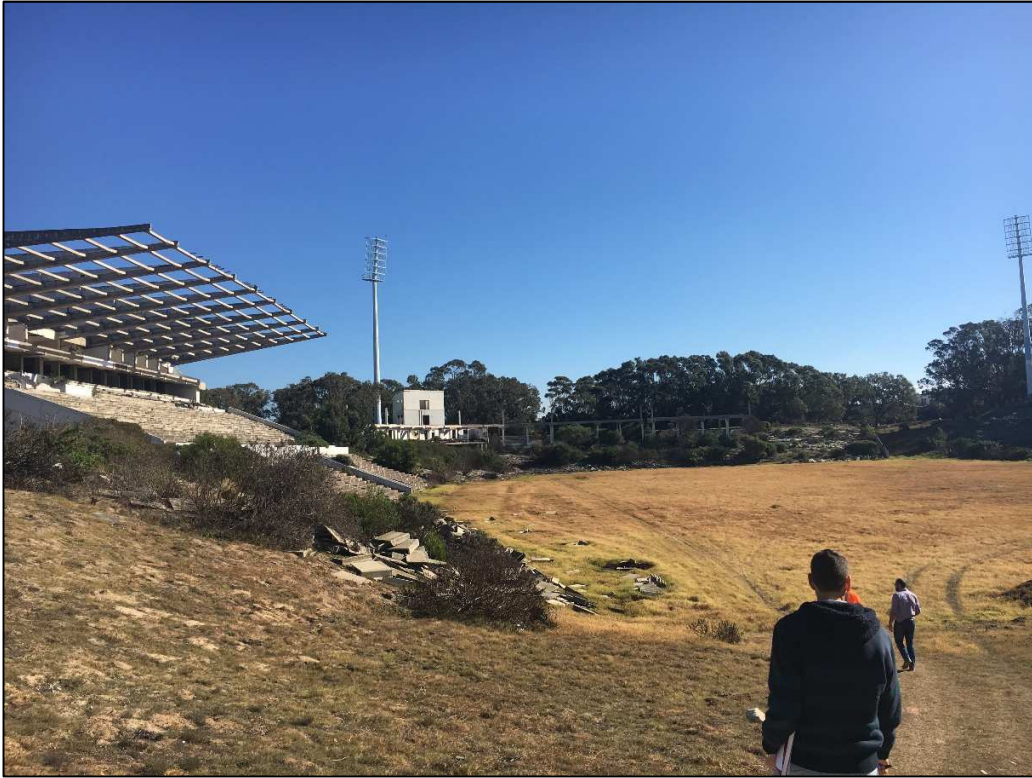
Photo 3: View of the corporate suites, located on the western side of the stadium facility.
