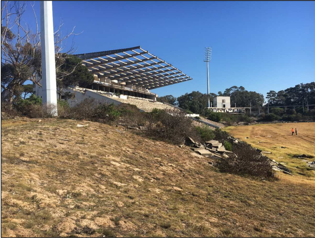
Photo 1: Showing the Main Pavilion and cantilever roof structure, located on the southern side of the stadium.
